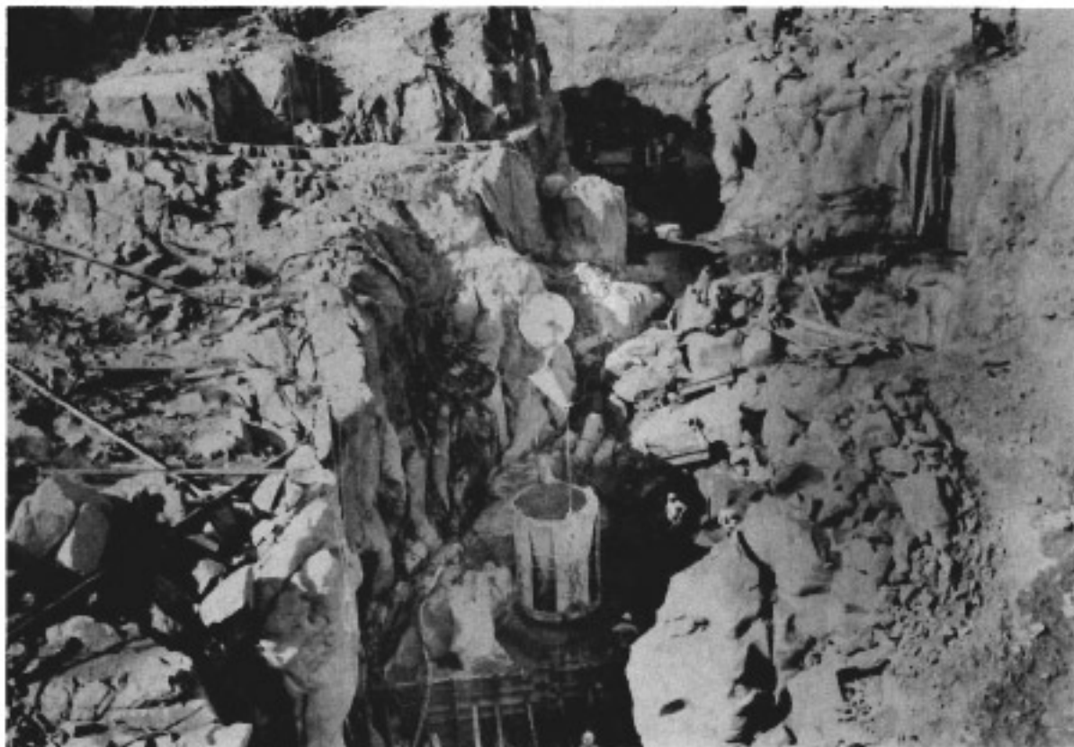
TULLOCH RIVERBED DURING EXCAVATION (Photo by Allen Holbrook, OID)
