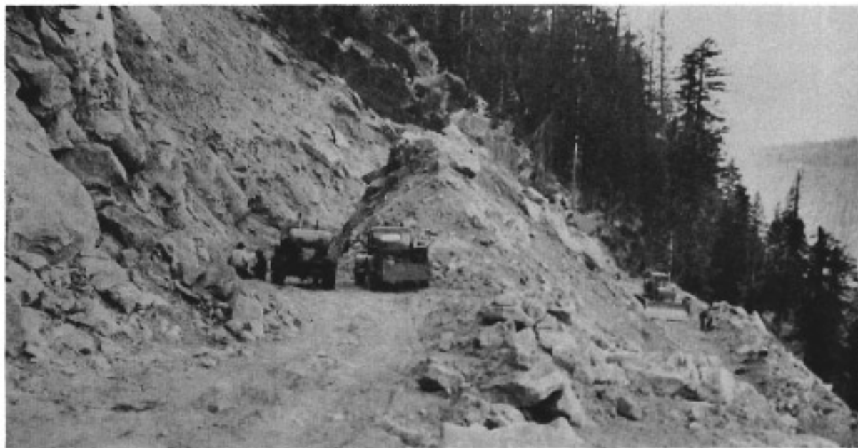
ACCESS ROAD INTO DONNELLS DAM SITE (Photo by Allen Holbrook, OI)
