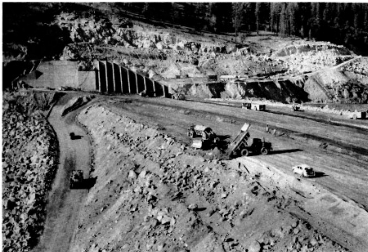
BEARDSLEY DAM DURING CONSTRUCTION (Photo by Allen Holbrook, OID)
