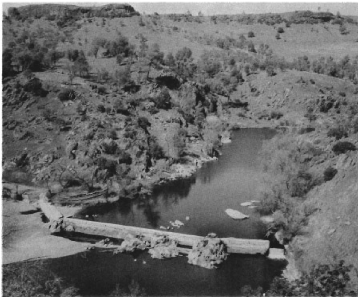
ORIGINAL TULLOCH DAM (Photo by Allen Holbrook, OID)
