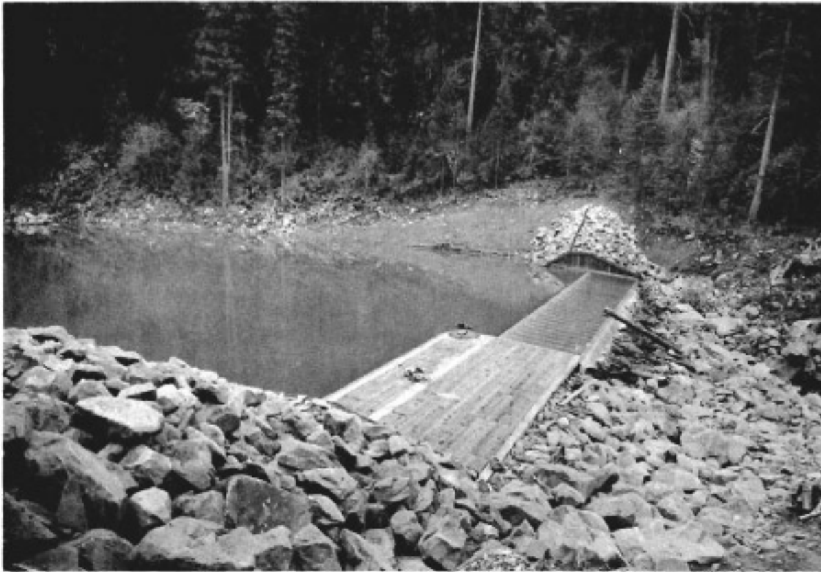
BEARDSLEY AFTERBAY DAM (Photo by Bob Hooe, Sonora)
