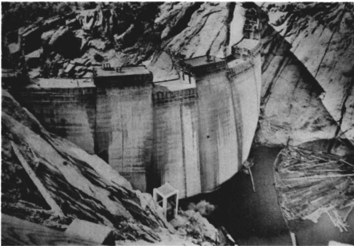
DONNELLS ARCH DAM DURING CONSTRUCTION (Photo by Bob Hooe, Sonora)
