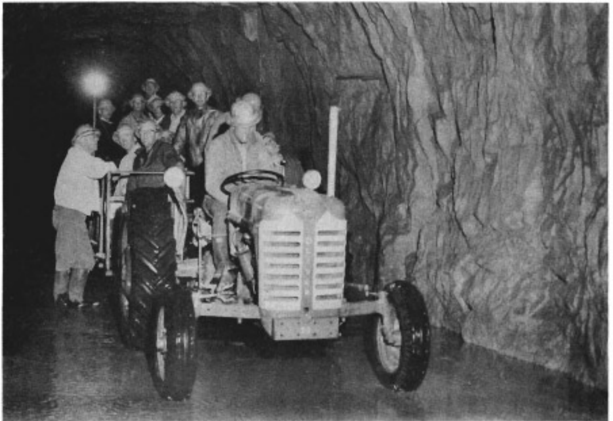
FINAL TUNNEL INSPECTION BY JOINT BOARDS - MAY 15, 1957 - DONNELLS (Photo by Bob Hooe, Sonora)
