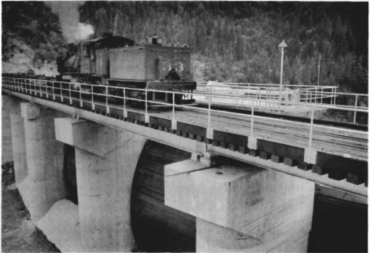
RELOCATED RAILROAD IN USE ACROSS BEARDSLEY SPILLWAY BRIDGE (Photo by Bob Hooe, Sonora)
