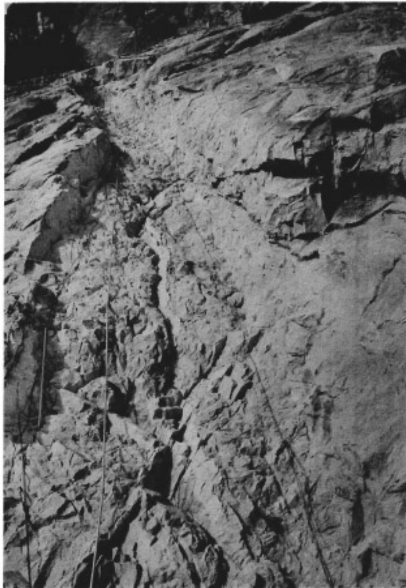
EXCAVATION FOR RIGHT ABUTMENT - DONNELLS DAM (Photo by Bob Hooe, Sonora)
