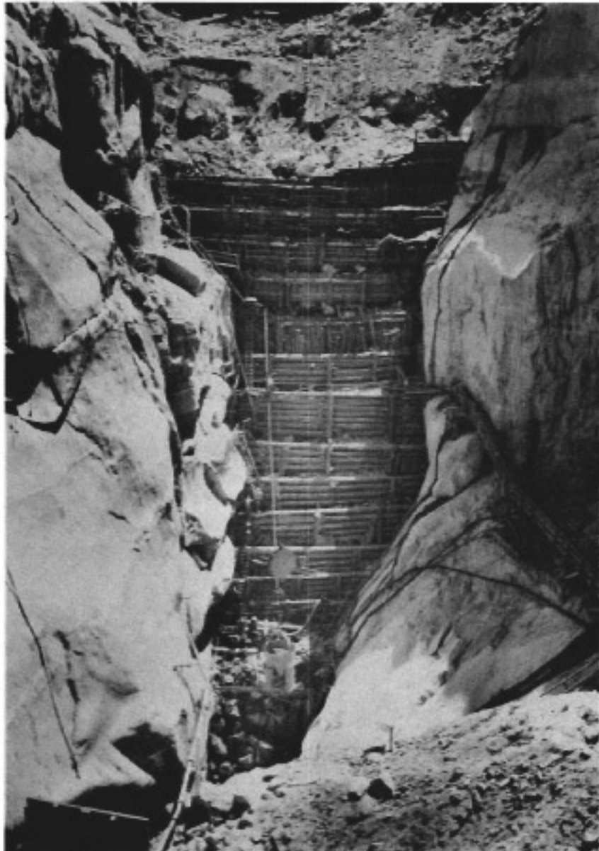
EXCAVATION OF GORGE - DONNELLS DAM (Photo by Allen Holbrook, OI D)
