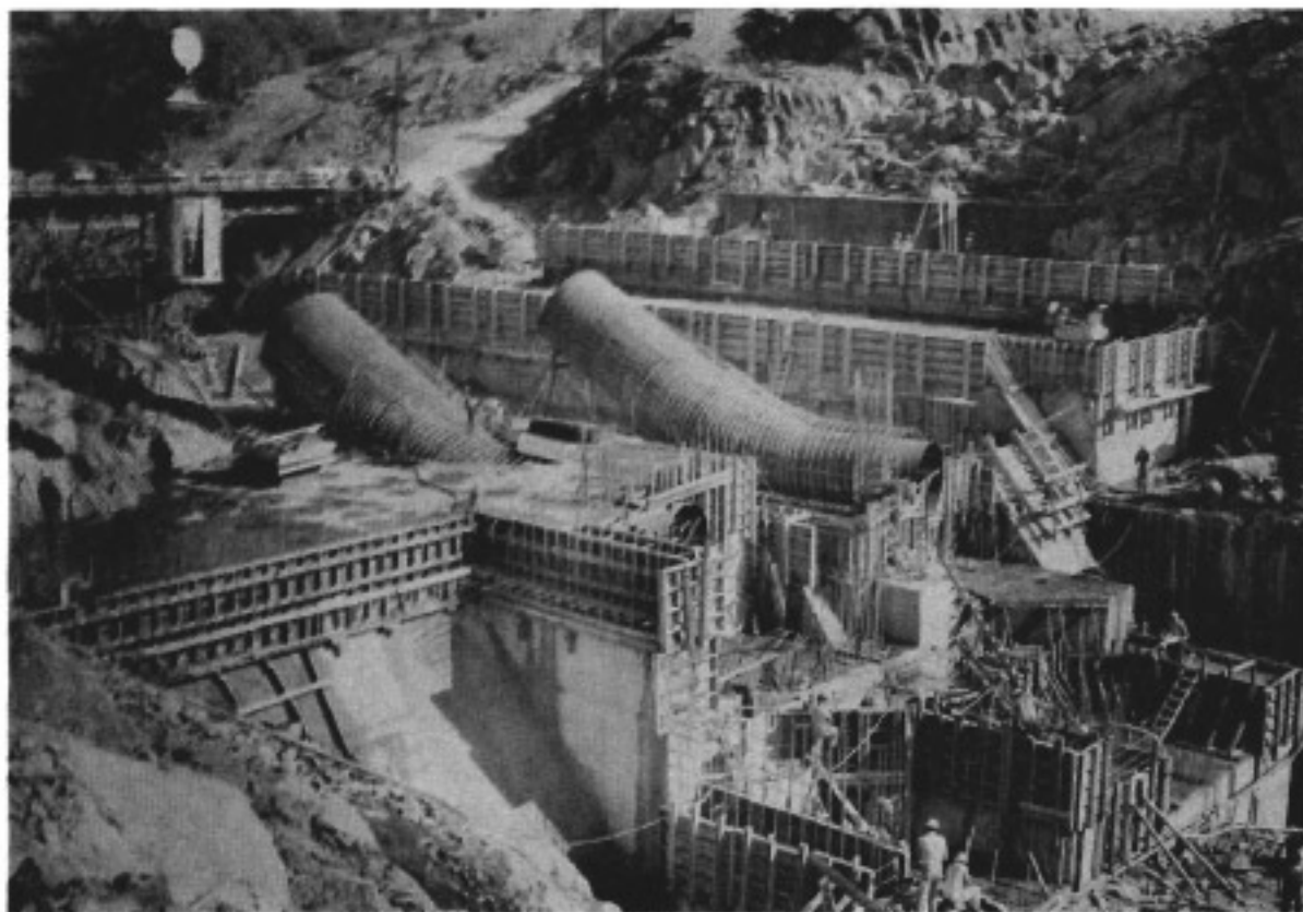
TULLOCH - DURING CONSTRUCTION (Photo by Allen Holbrook, OI D)
