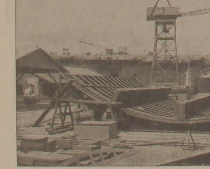
Assembling one of the dam gates at Todd Plant
