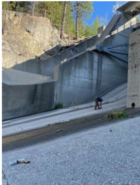
Beardsley Spillway Maintenance
