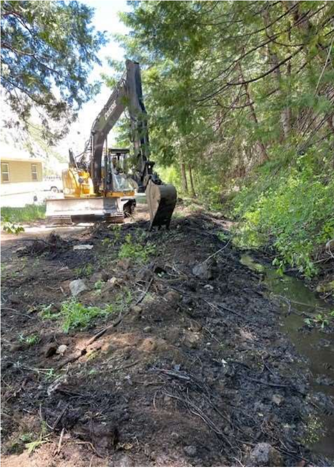
Donnells Cottage Drainage Restoration
