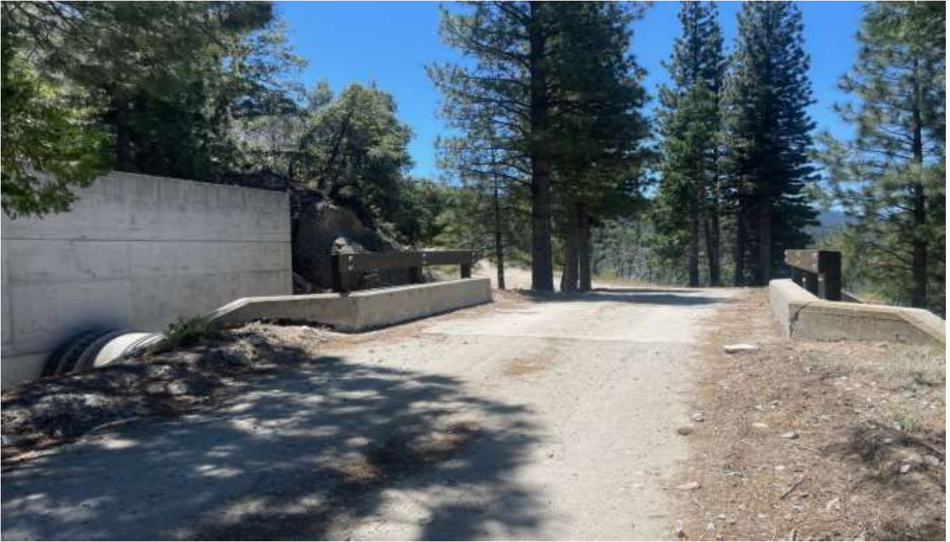
Penstock Bridge Guardrail
