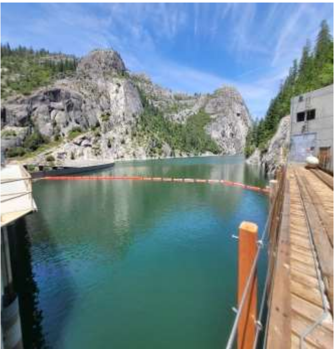
Donnells Dam Log Boom
