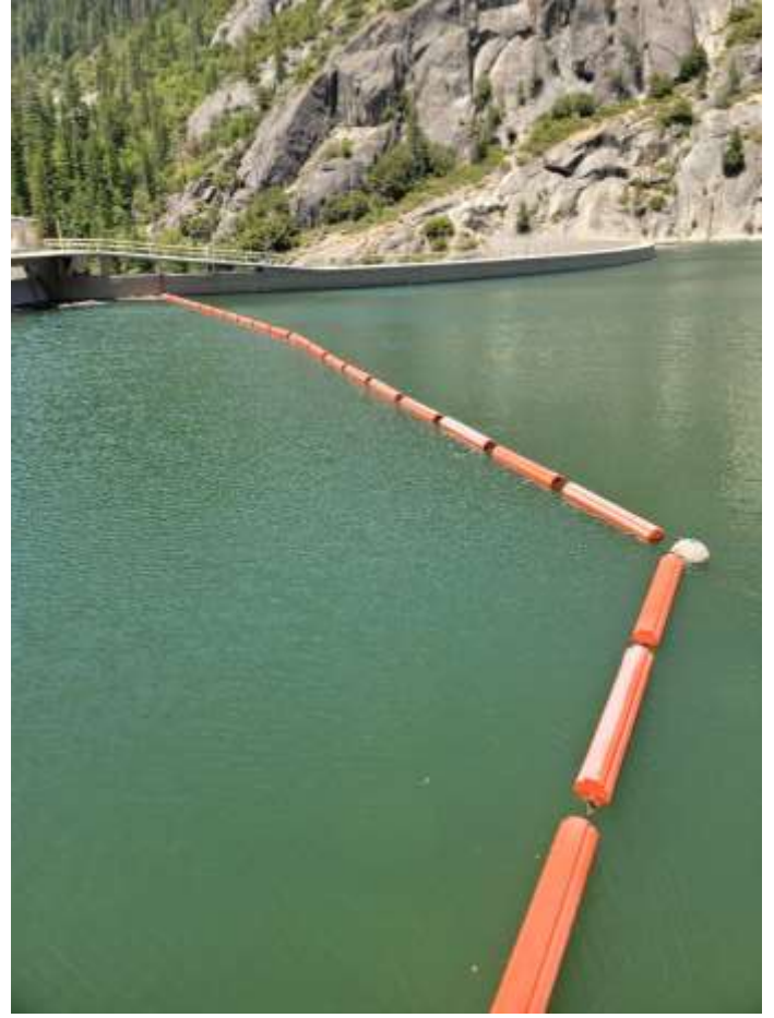
Donnells Dam Log Boom
