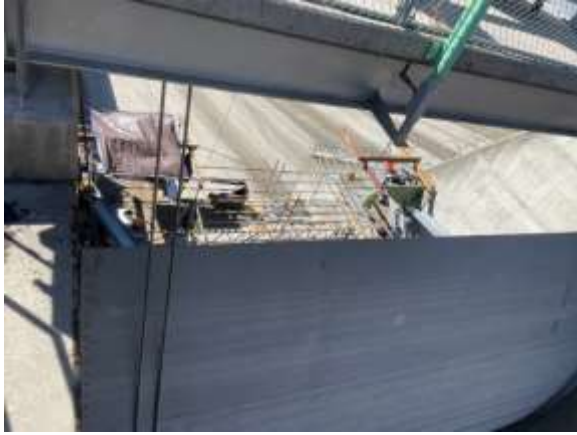
Figure 1: Beardsley trunnion pin progress
