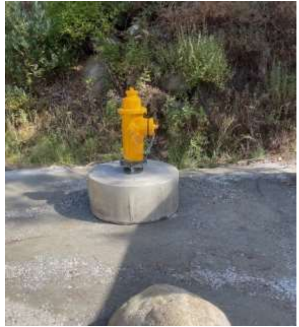
Figure 4: DPH hydrant replacement
