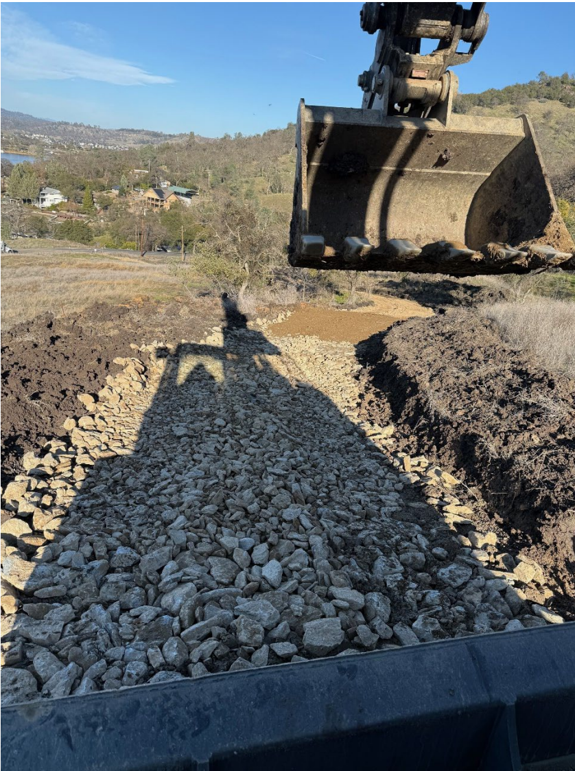
Water Tank Road Repair at Tulloch
