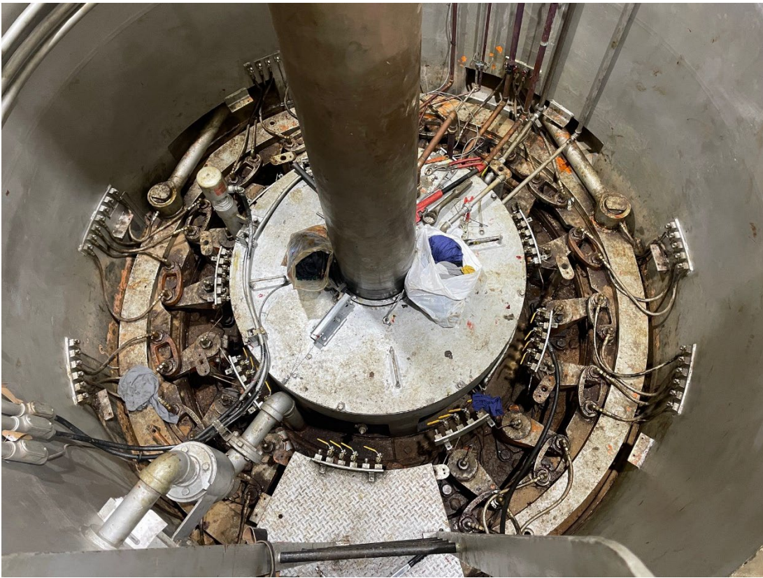
Maintenance of Wicket Gates and Linkage- Tulloch
