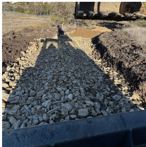
Figure 1: Tulloch raw water road material placement
