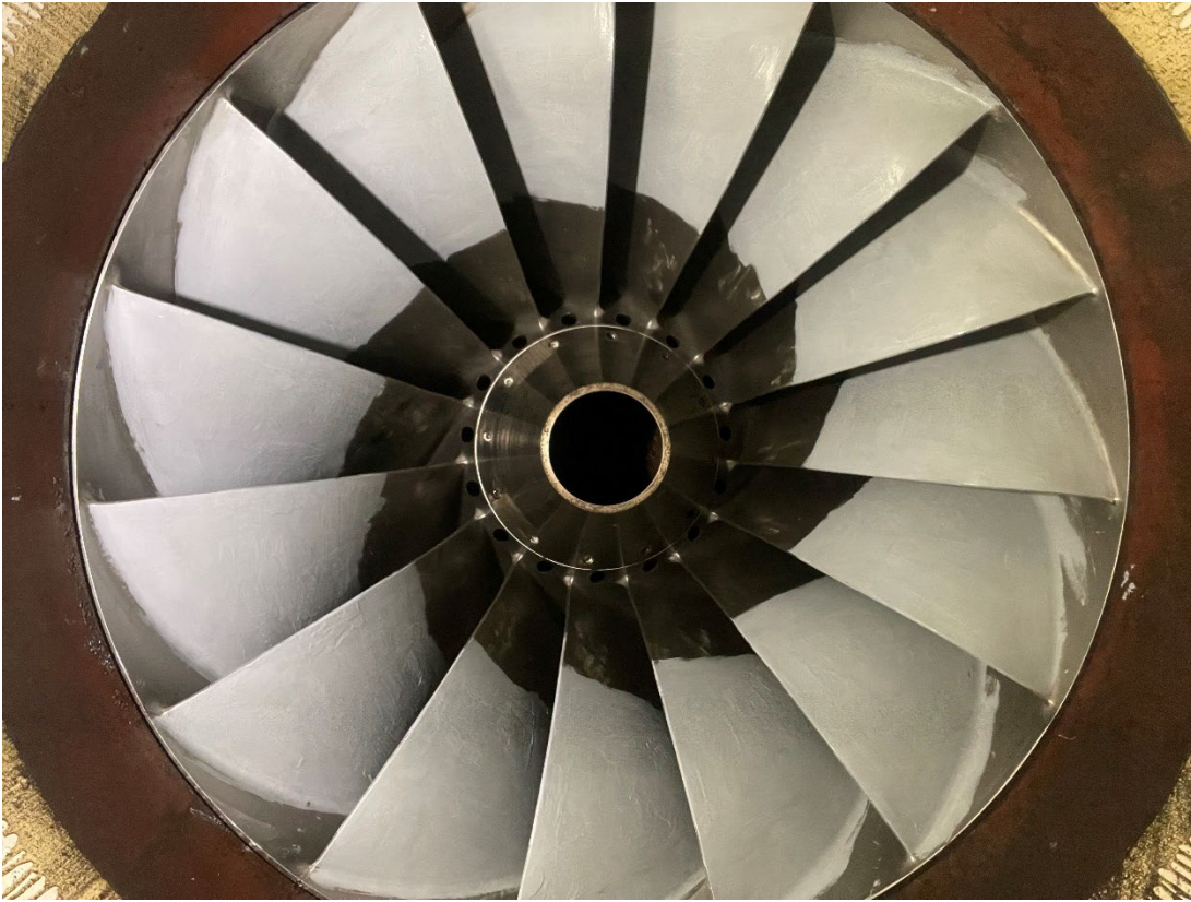
TPU Unit 2 Wheel Repairs
