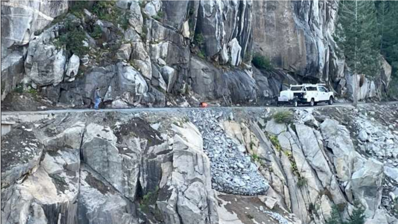
FEMA Site 5- Sink Hole Repair
