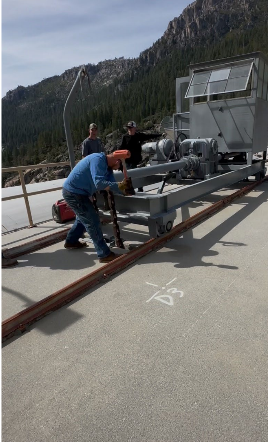
Setting the chain after bump testing the gate under hand power
