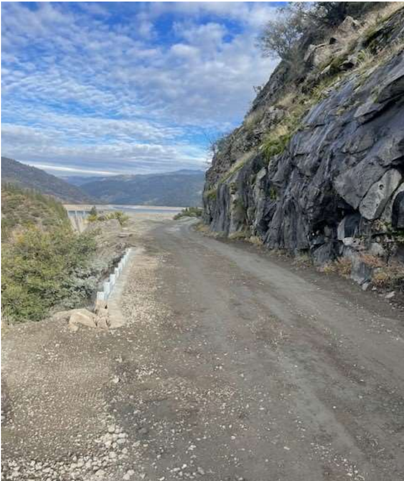
FEMA Site 2 near Beardsley Dam
