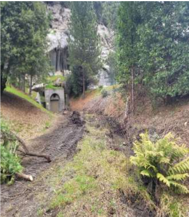
Sandbar Tunnel Access – Before
