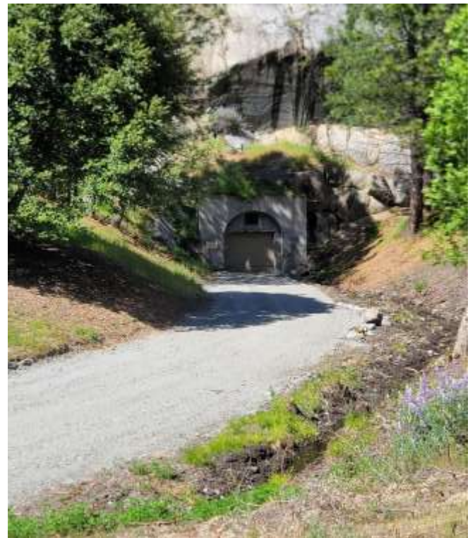
Sandbar Tunnel Access - After
