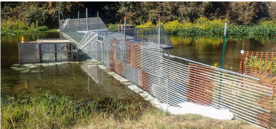
Figure 3. Tuolumne River weir following installation.
