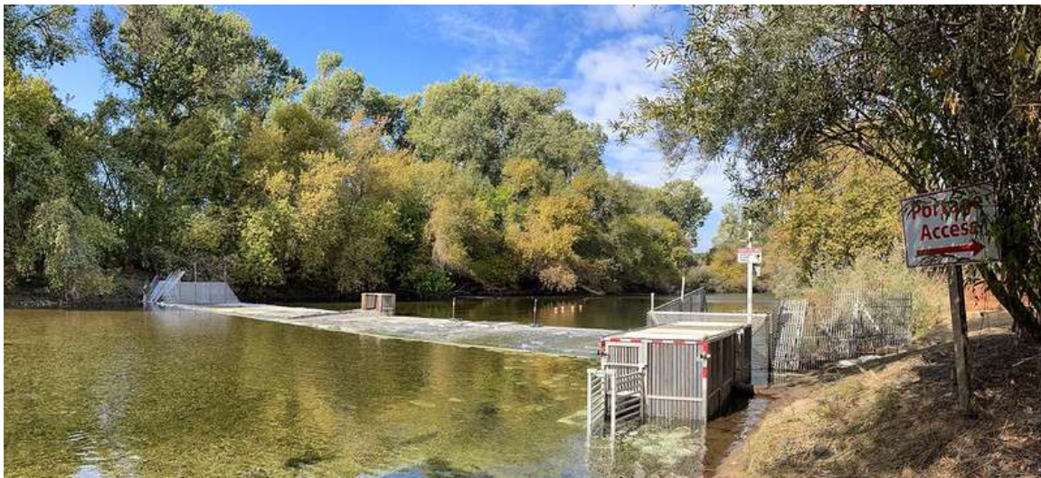
Figure 1. Stanislaus River weir following installation.
